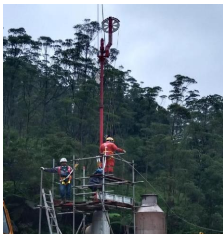
Fig. 9. Lubricator with hydraulic stuffing box and crown pulley on the wellhead of Well-A.
